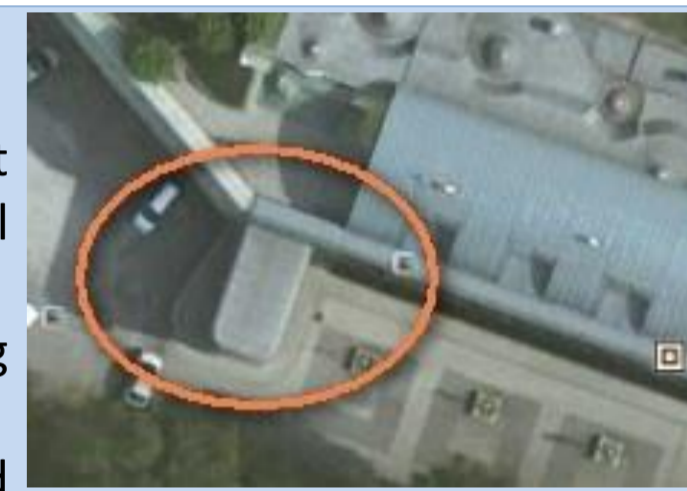
Fig. 10. The caponier of the Węgrzce Fort (source: Google Maps).
